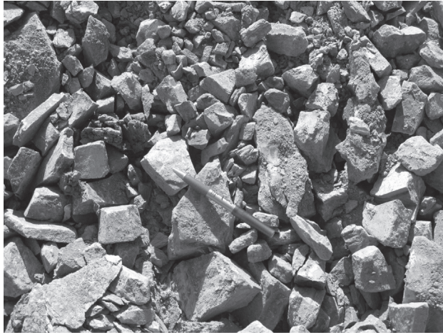
Figure 7 - Lechago dam. Detail of rockfill.
