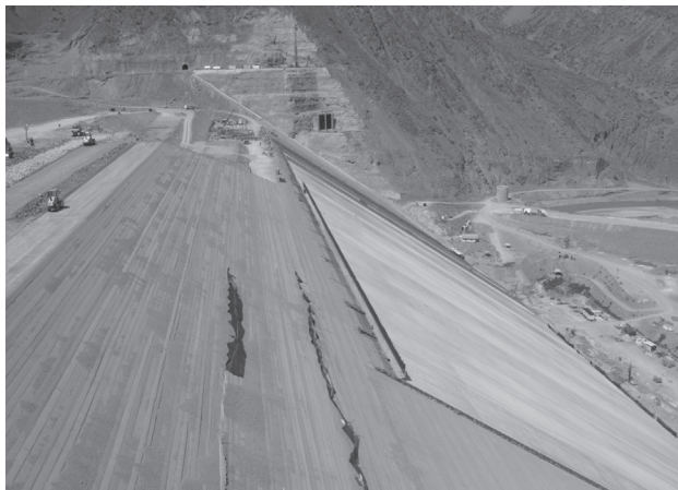
Figure 2 - Caracoles dam under construction (2007). San Juan, Argentina.
