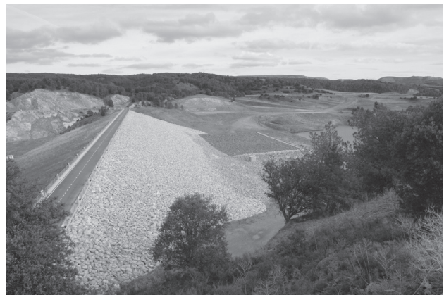
Figure 5 - Lechago dam, Teruel, Spain. February 2008.
