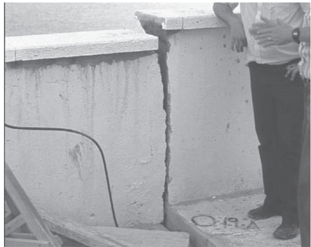
Figure 10 - Collapse settlements of rockfill in Calanda dam.
