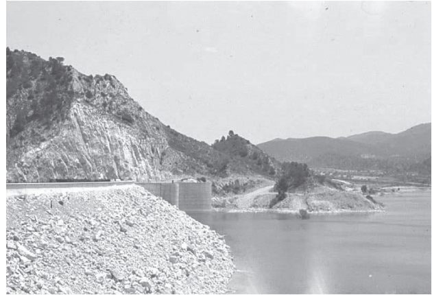
Figure 9 - Calanda dam, Teruel, Spain.
