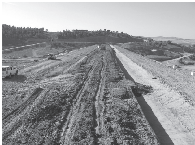
Figure 6 - Lechago dam. Core, filters and rockfill shoulders.
