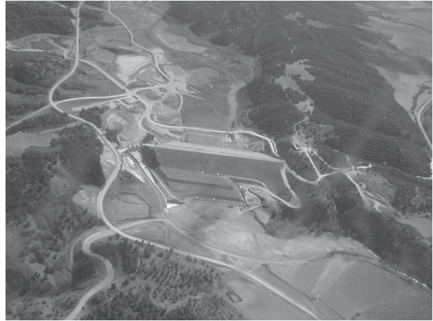
Figure 4 - Lechago dam, Teruel, Spain. Aerial view. February 2008.
